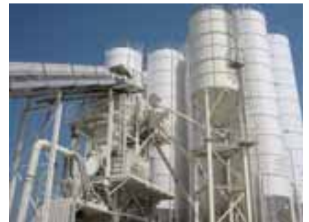
4.5 cbm twin-shaft compulsory mixers by IME are used in both plants. Each plant is equipped with 9 cement silos.
